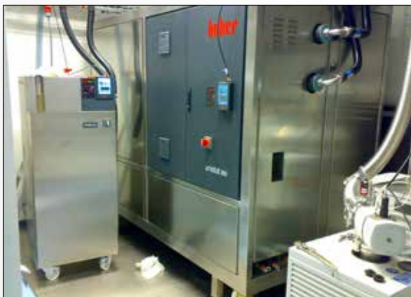
A Unistat 950w controls the temperature of the vacuum chamber, another Unistat 915w the table for the experiments
